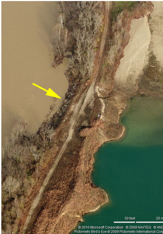
Figure 18. Site of the 2003 breach (yellow arrow) of berm separating quarry from Great Miami River (see Figure 12 ).
