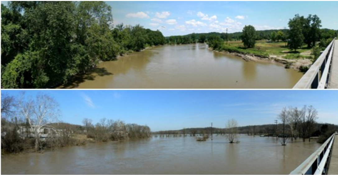
Figure 34. Views of Great Miami River looking upstream from the Miamitown bridge: high-normal discharge, July 1, 2008 and flood discharge March 20, 2008 (bottom)
