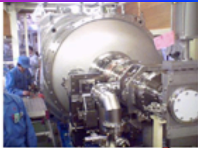
Crab cavities will be installed and tested with beam in 2006.
