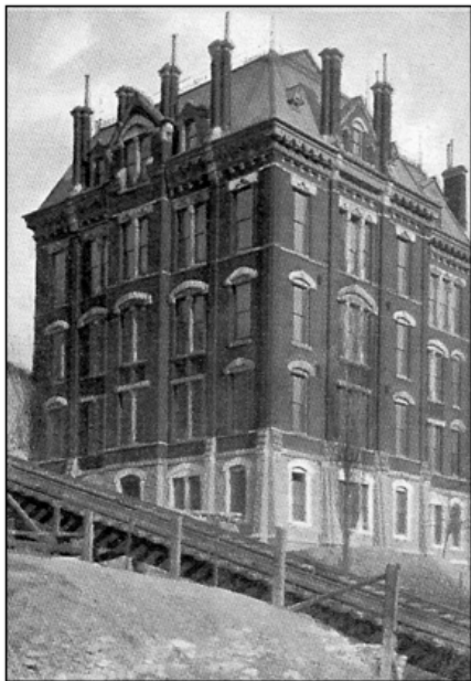
Figure 6. The tracks to the incline that ran along the west side of the original university building.
