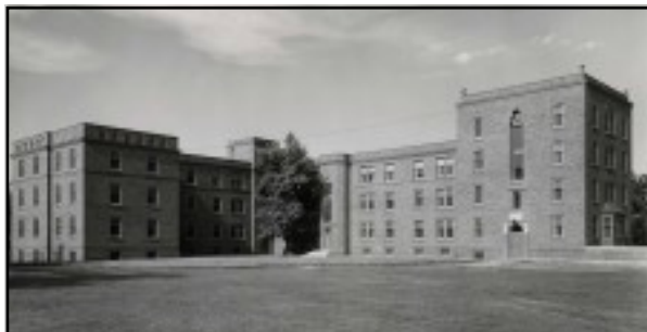
Figure 5. A fuzzy snapshot of the old dormitories at Augsburg College. Dating from 1938 and originally known Sverdrup-Oftedal Memorial Hall, their current fate could not be determined from the College website.
