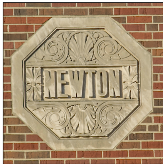
Figure 6. One of the six octagonal medallions that decorate the cornice of the 1932 UC physics building.
