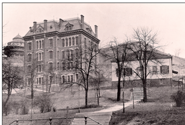
Figure 3. The University of Cincinnati as it appeared during Warder's association with the school. Located on the steep slope of the Vine Street Hill, roughly at the point where Clifton Avenue takes a sharp turn to the east, the chemistry laboratory was originally located in the basement of the brick building on the left. The University moved from this site to its present location near Burnet Woods in 1895.
