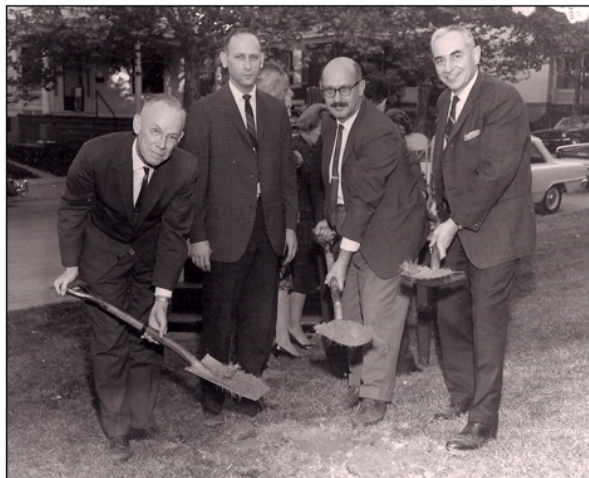
Breaking ground for the new chemistry building in 1964. From left to right: Tom Cameron, Fred Kaplan, Hans Jaffé, and Milt Orchin.
