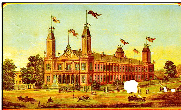
Figure 5. A damaged colored lithograph of the original Exposition Hall where the Cincinnati Industrial Exposition of 1870 was held. Made of wood, it was torn down a few years later and replaced with the current brick structure known as Springer or Music Hall.
