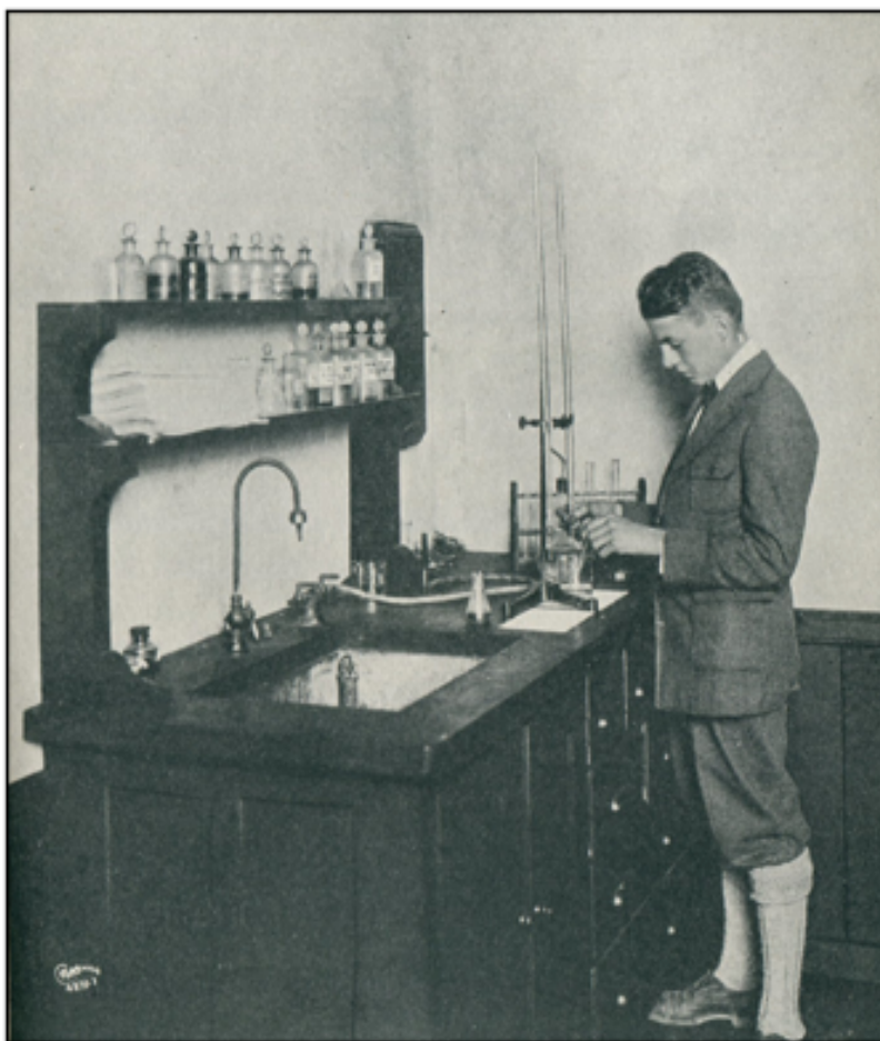
Determining the strength of an acid by titration.
