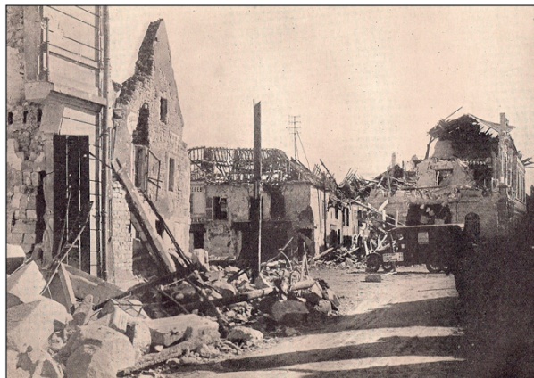
Figures 27-28 (below). Two views of the ruins of Fismes France after its capture on 4 August 1918.
