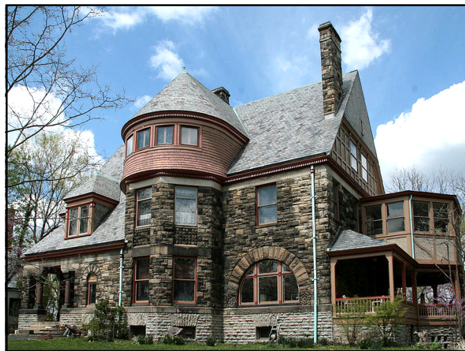
Figure 3. The Lloyd mansion at 3901 Clifton Avenue, now listed on the National Register of Historic Homes.
