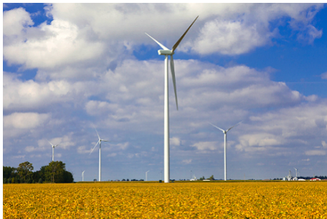
Blue Creek Wind Farm in Ohio. (Courtesy Iberdrola Renewables)
