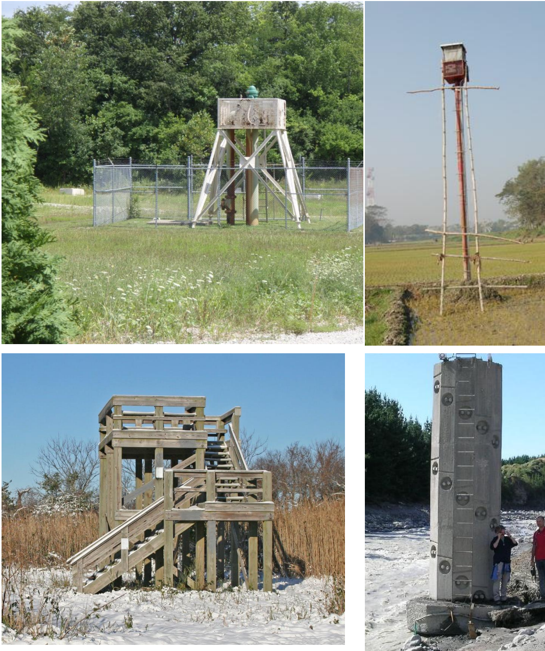
Figure 13. Example of simple platforms of types that could be used to elevate well-head above flood level. The elevated platform for GMWO would be designed in consultation with Hamilton County Park District.
