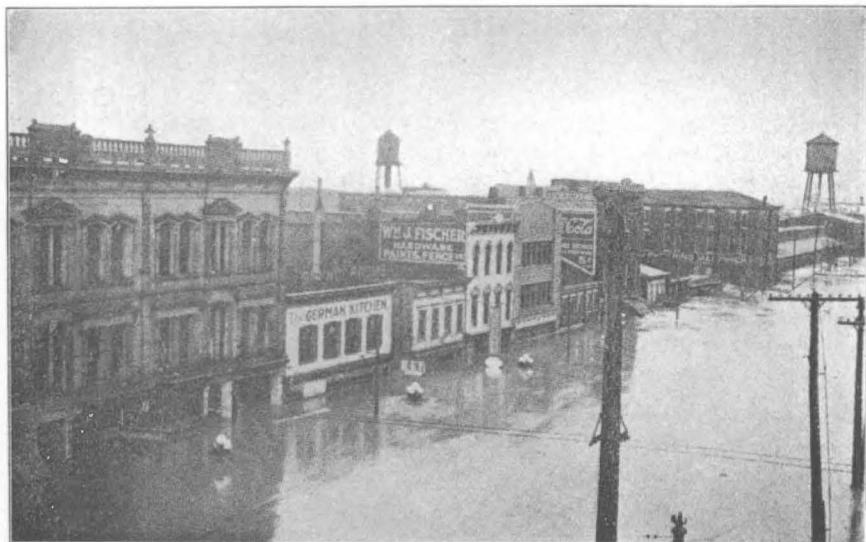
A.—Flood at Hamilton, March 26, 1913. (U. S. Geol. Surv. Water Supply Paper 334.)
