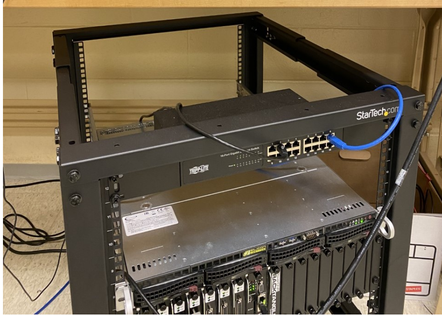
Figure 8: A picture of the UEI crate that connects the backpack to the GCP.
